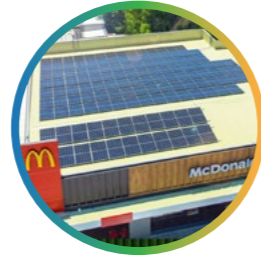
Installation of solar panels
