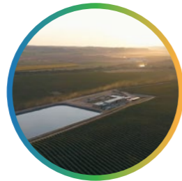
Rainwater recovery system
