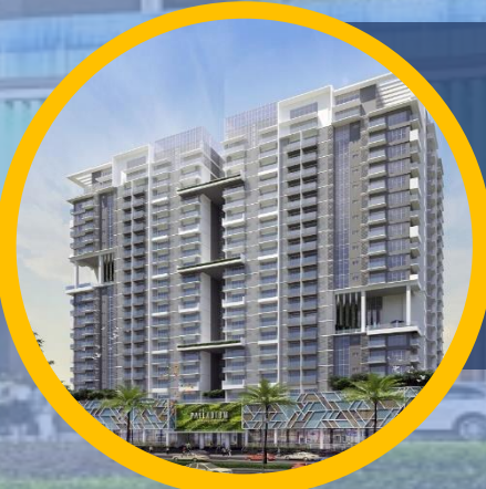
📍 Iloilo Business Park The Palladium (North & South Wing)
